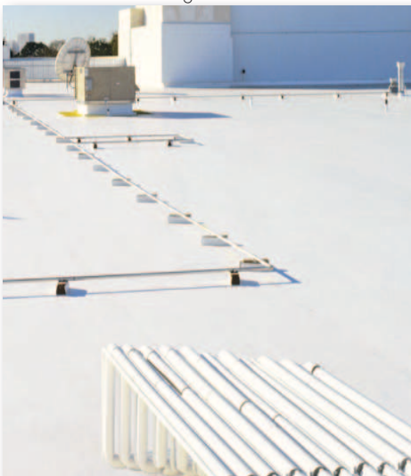
Shown: Reflective Roofing
