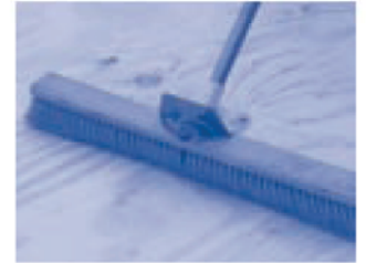
Step 1 Sweep dirt from substrate
