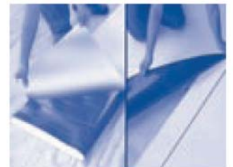
Step 3 Remove release film (left) and adhere membrane (right)
