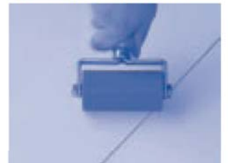
Step 4 Roll edges, seams, field of roof
